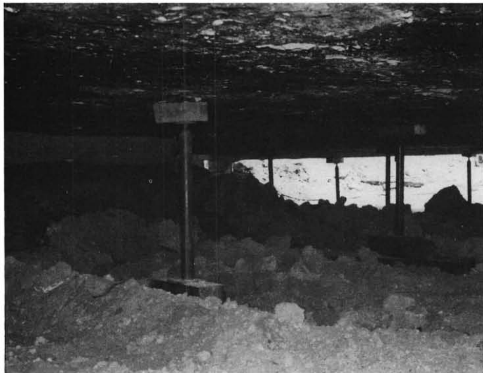
... to allow access to insert temporary supports for the slab.
