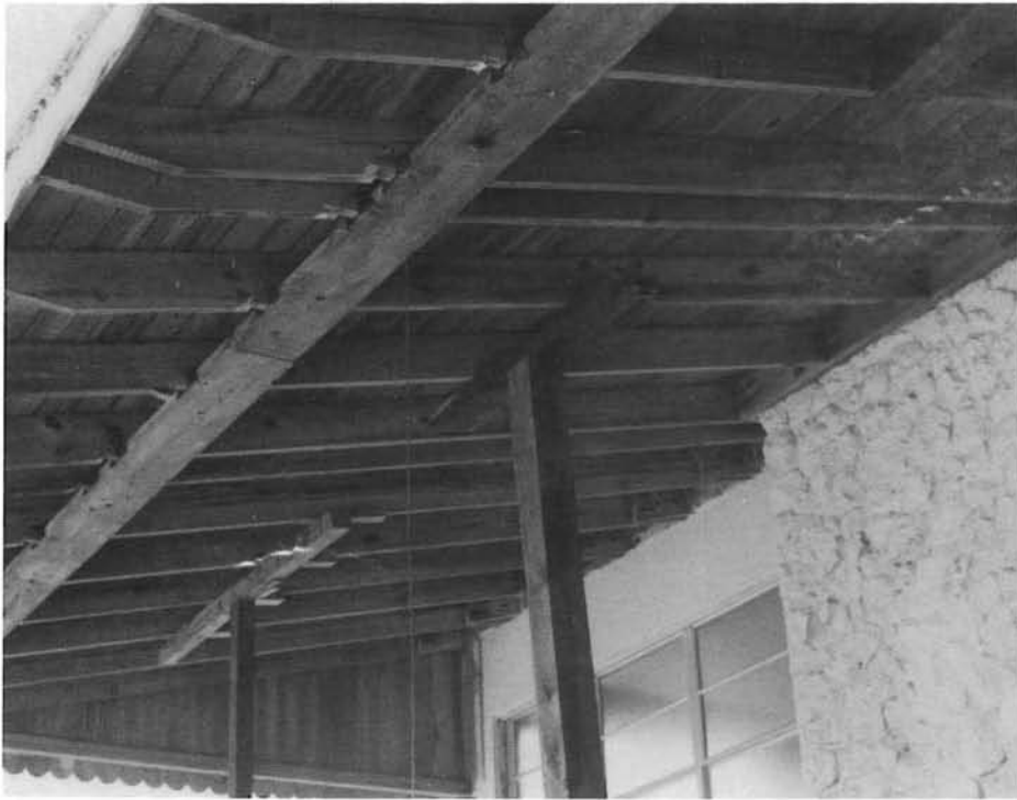
The wooden porch roof is temporarily supported...
