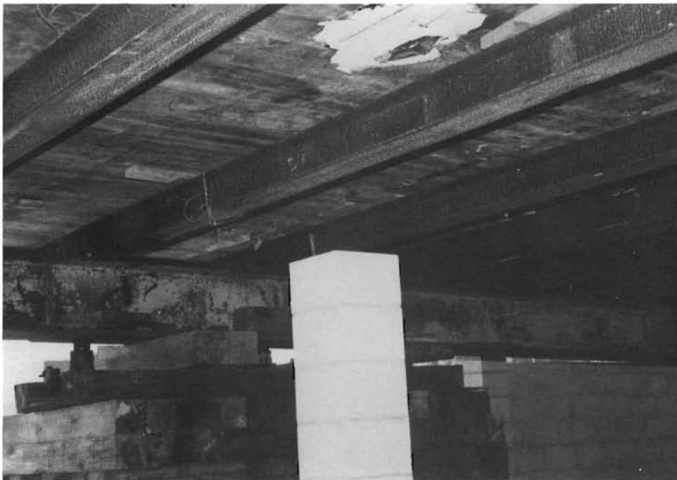
...cut away using an air saw.
