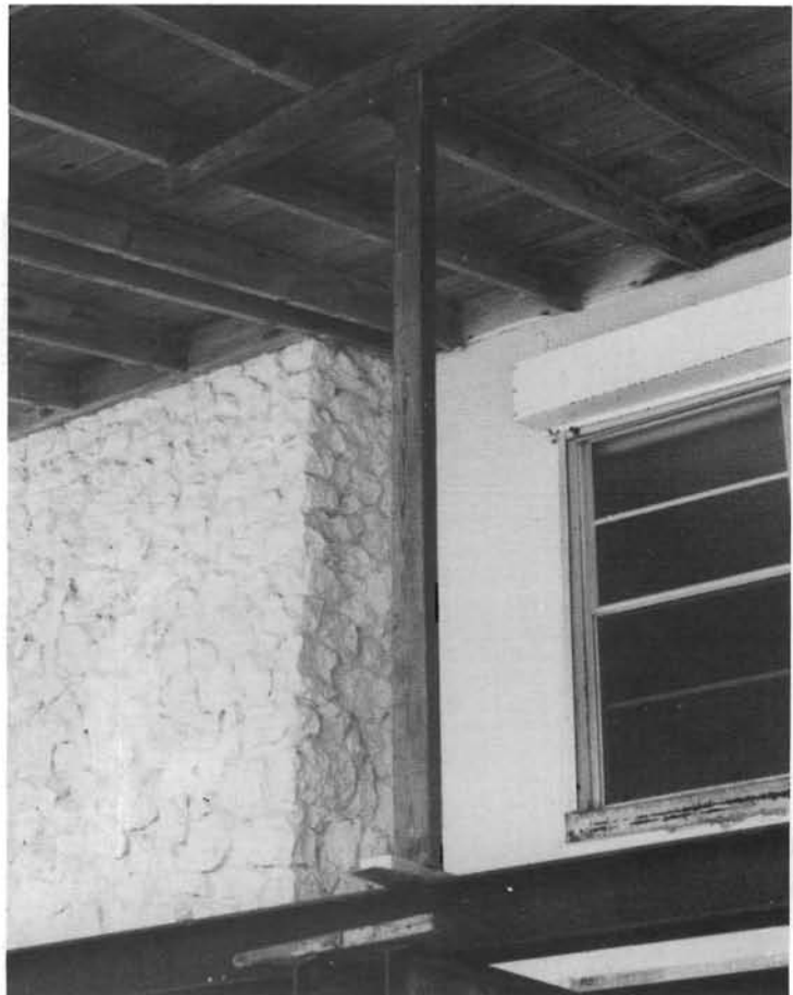
...from the steel framework
