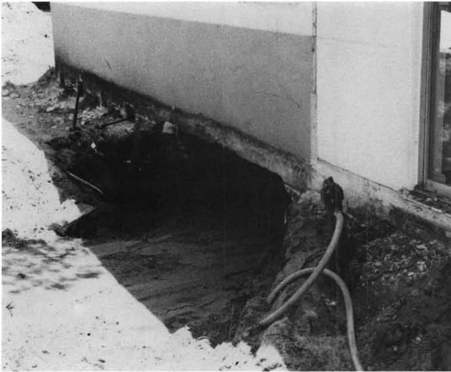
Excavation and tunneling have been carried to a sufficient depth...
