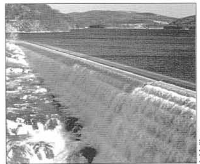
Figure 17 Though still meeting safe drinking water standards, some of New York City's 19 reservoirs have been adversely impacted by runoff and other non-point source pollution in recent years. Protecting floodplain resources throughout the watershed, such as by preserving and restoring vegetated riparian buffers, will help to maintain and enhance the drinking water for over 9 million people.
