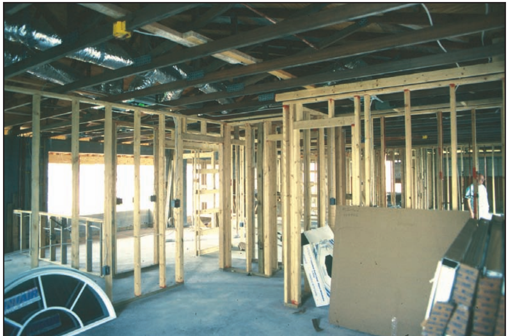
Figure 30 Interior partition walls and utilities are added.
