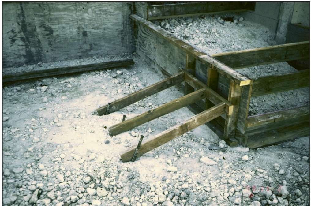
Figure 33 Wood framing for a new concrete staircase that will provide access to the elevated floor.
