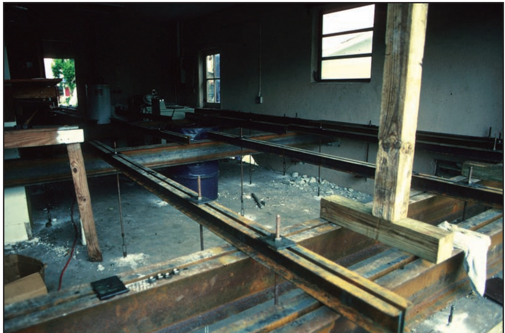
Figure 79 The anchors and hangers connect the slab securely to the beams, enabling the beams to raise the slab along with the rest of the house.
