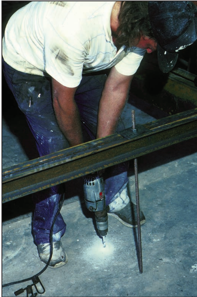
Figure 77 ... install anchors ...
