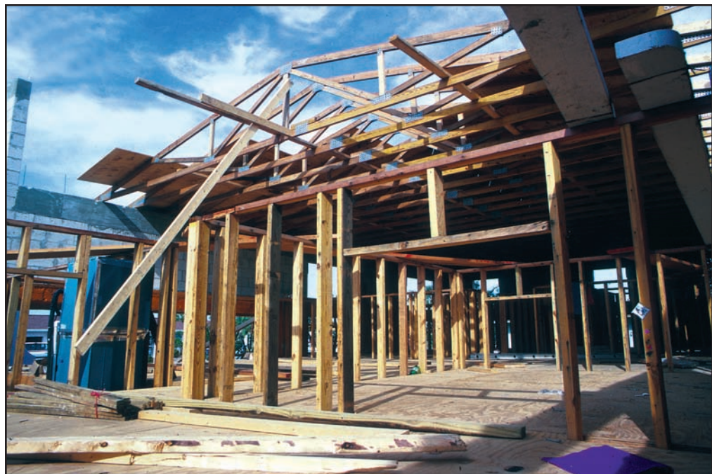
Figure 69 Wood framing is used for the new second story.
