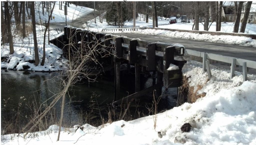
Figure 5.4.4-8. Carol Drive wood timber bridge
